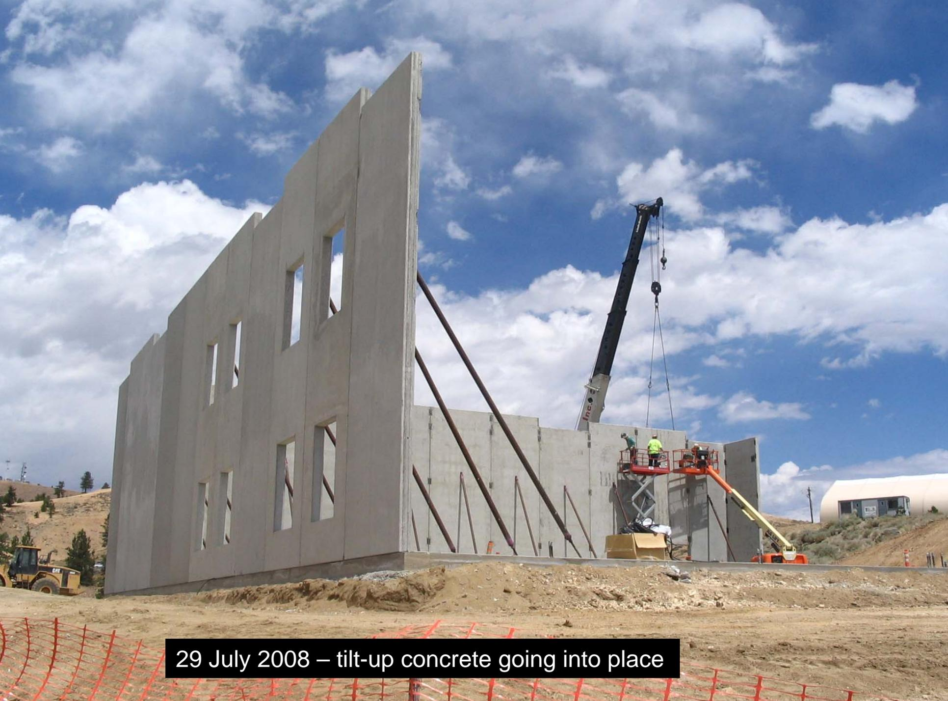
29 July 2008 – tilt-up concrete going into place
