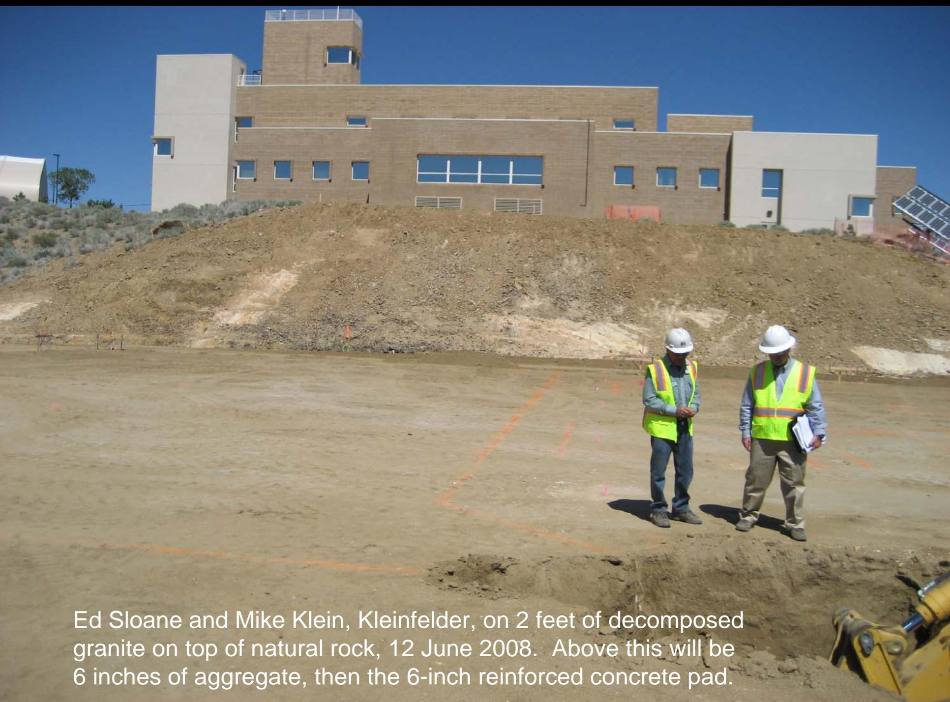
Ed Sloane and Mike Klein, Kleinfelder, on 2 feet of decomposed granite on top of natural rock, 12 June 2008. Above this will be 6 inches of aggregate, then the 6-inch reinforced concrete pad.
