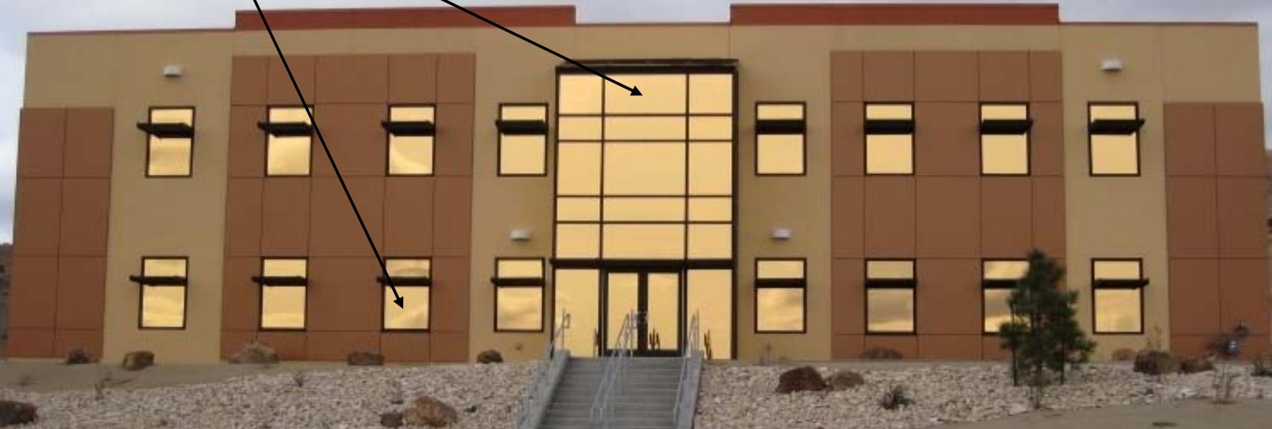
**[26 windows x (4 ft x 6 ft)/window + 20 ft x 20 ft for vestibule] x (1 m/3.2808 ft)<sup>2</sup> x [1.73 x 10<sup>-8</sup> m thick gold coating] x 19.3 metric tons/m<sup>3</sup> x 3.21507 x 10<sup>4</sup> troy ounces/metric ton = **1.02 troy ounces of gold** on these windows.**
