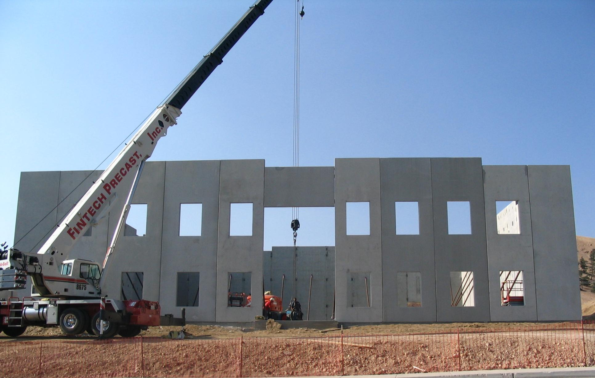
30 July 2008 – tilt-up concrete going into place
