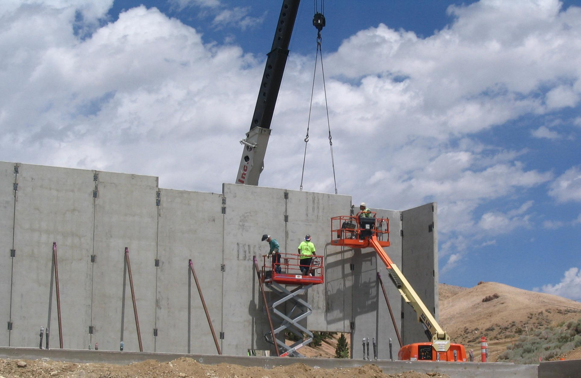
29 July 2008 – tilt-up concrete going into place
