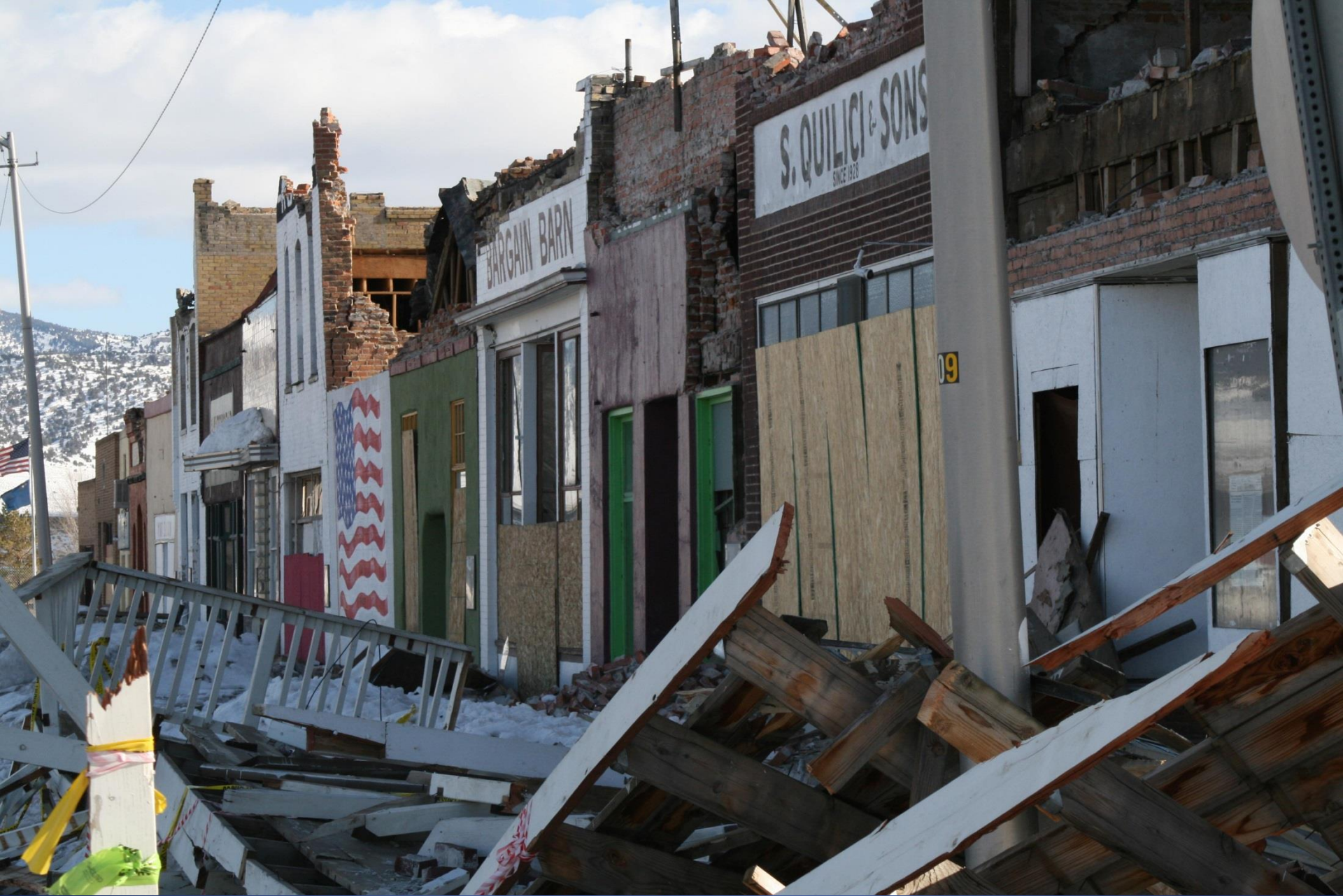
2008 Wells, Nevada Earthquake Damage – Front Street
