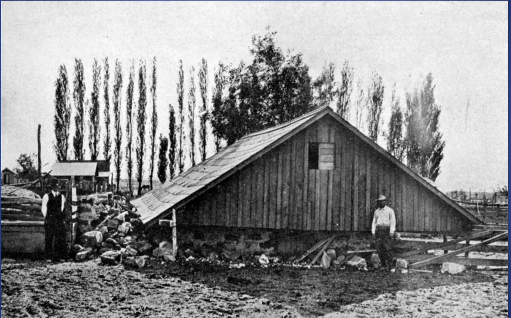
View south – men stand where walls were
