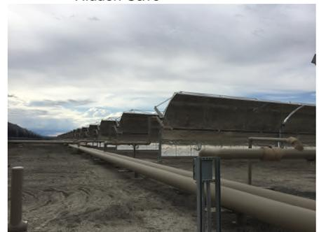
Concentrating Solar Assist for Geothermal Plant
